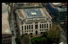
areas, with the larger hole-sized product providing the correct level of ventilation for the Air Handling Units, and the smaller hole sizes of the mini mesh providing additional privacy in other areas of the roof to minimize the impact on the historic views of St Paul's. Nonconductive, lightweight and requiring minimal maintenance, the Dura Grating panels were supplied with powder coated fixing clips and hinged access panels, and offered the perfect strengthto-weight ratio for the project.
