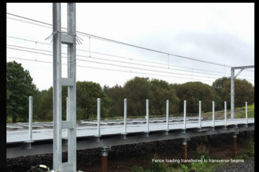
Fence loading transferred to transverse beams
